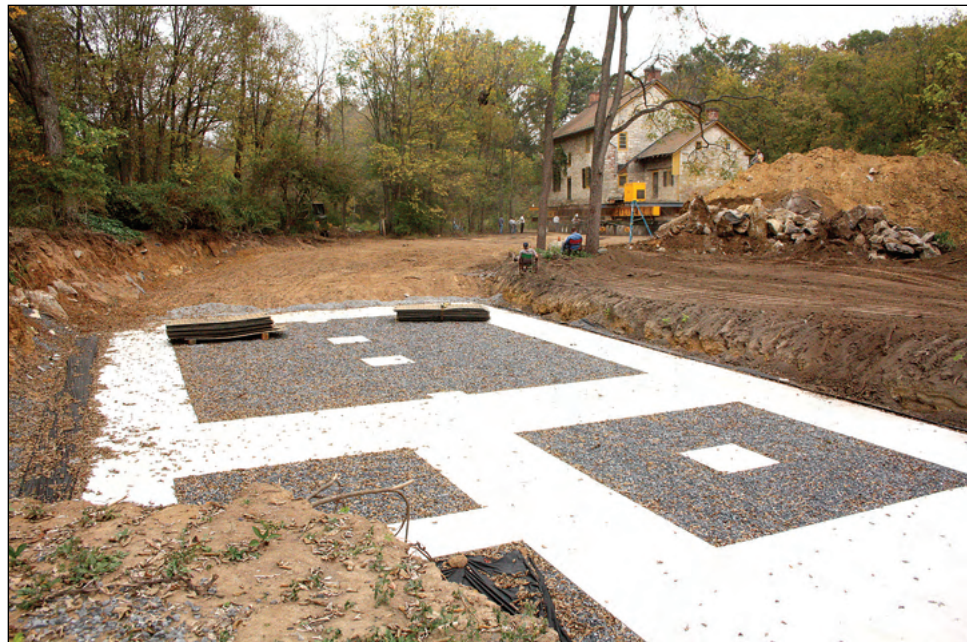
Figure 6-1. New foundation is being prepared (photo courtesy of Wolfe House Movers).
