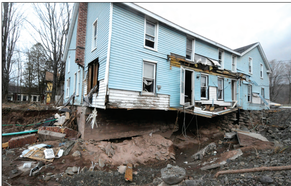
Figure 3 13. Many homes in the Town of Prattsville, NY, were slated for demolition during the recovery effort following Hurricane Irene.
