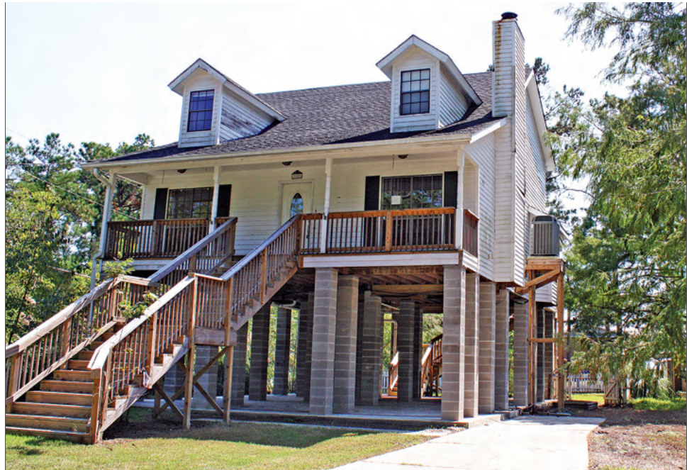
Figure 5-8. House in Zone A was detached from its slab foundation (which remains) and elevated on masonry piers. The floor system is supported by new wood joists (Mandeville, LA).
