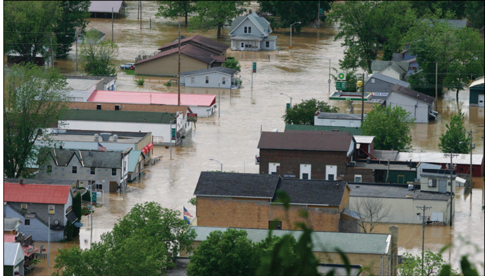
Figure 2-3. These homes in Gays Mills, WI, were inundated by riverine flooding during the Midwest floods of 2008.
