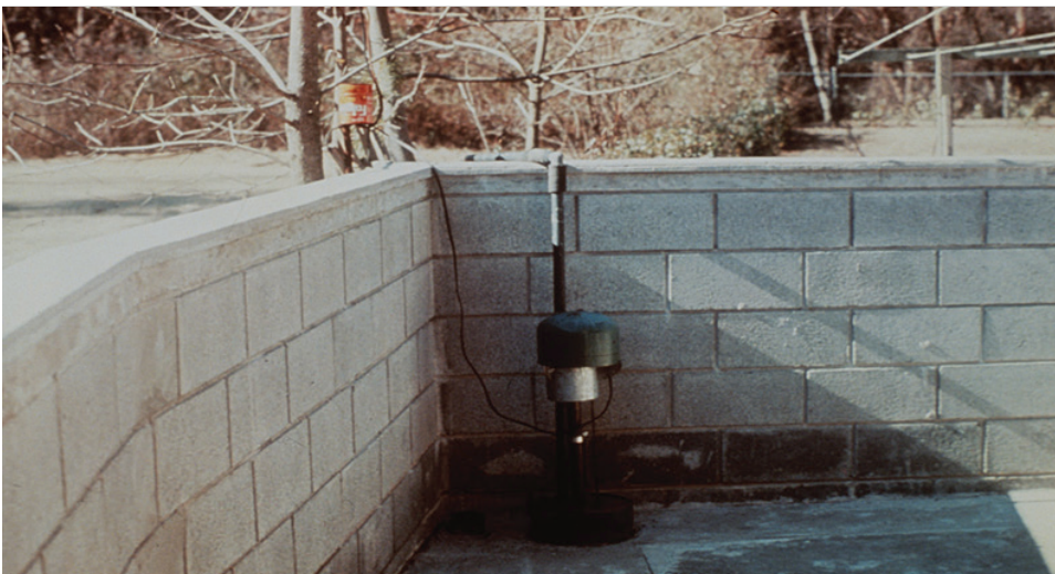
Figure 8-6. Small patio floodwall with sump pump.
