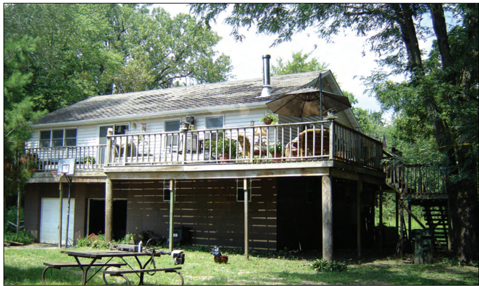
Figure 5-2. This home in Cedar Falls, IA, was elevated one full story. The garage and storage area are at the home's original elevation.
