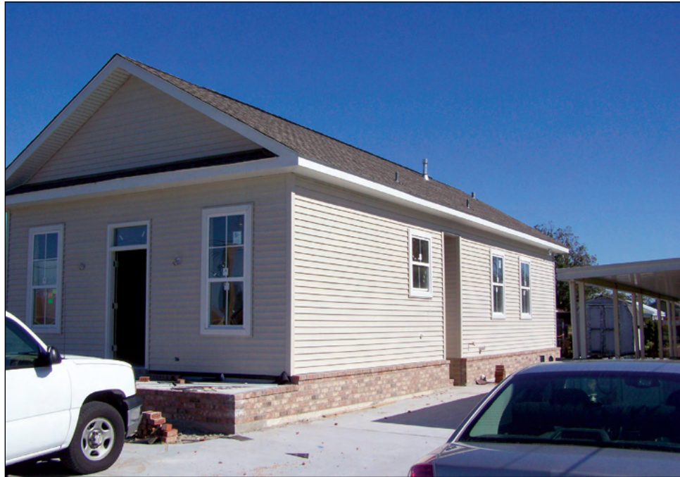
Figure 6-9. Typical mitigation reconstruction project.
