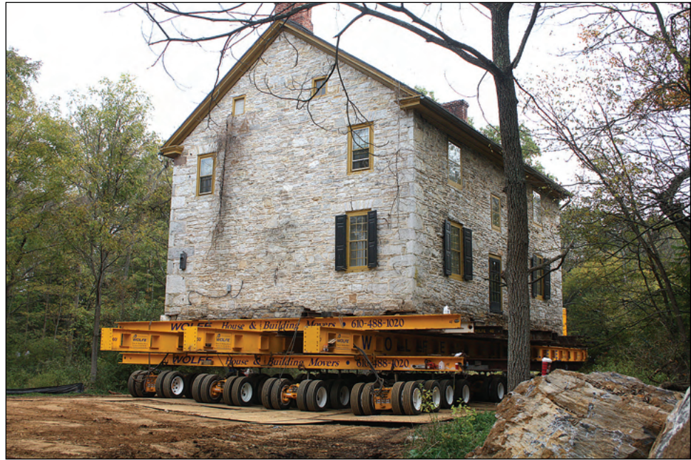
Figure 6-7. The move to the new site begins (photo courtesy of Wolfe House Movers).
