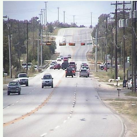
Figure 6–7, Roadway Utilizing Varying Methods of Access Management
