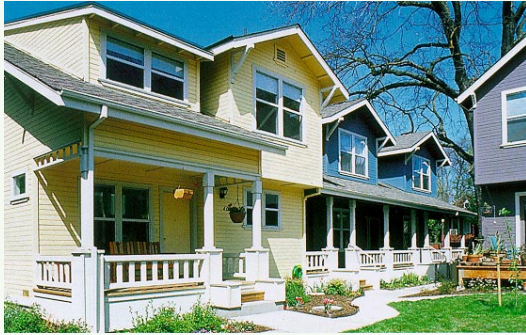
Duplex Units, Southside Park in Sacramento, California
