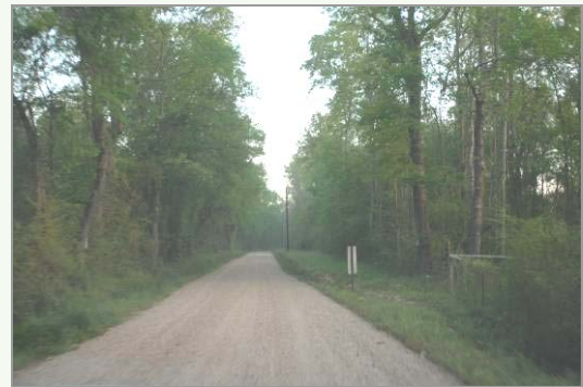
Figure 3-11, Gravel Road in Tangipahoa Parish
