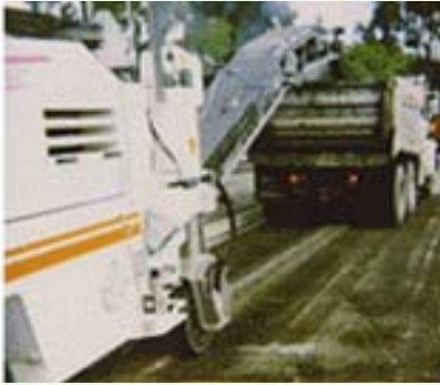
Figure 6-6, Resurfacing of Roadway
