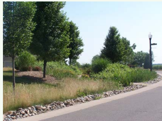
Figure 3–18, Road Ditch Bioswales
